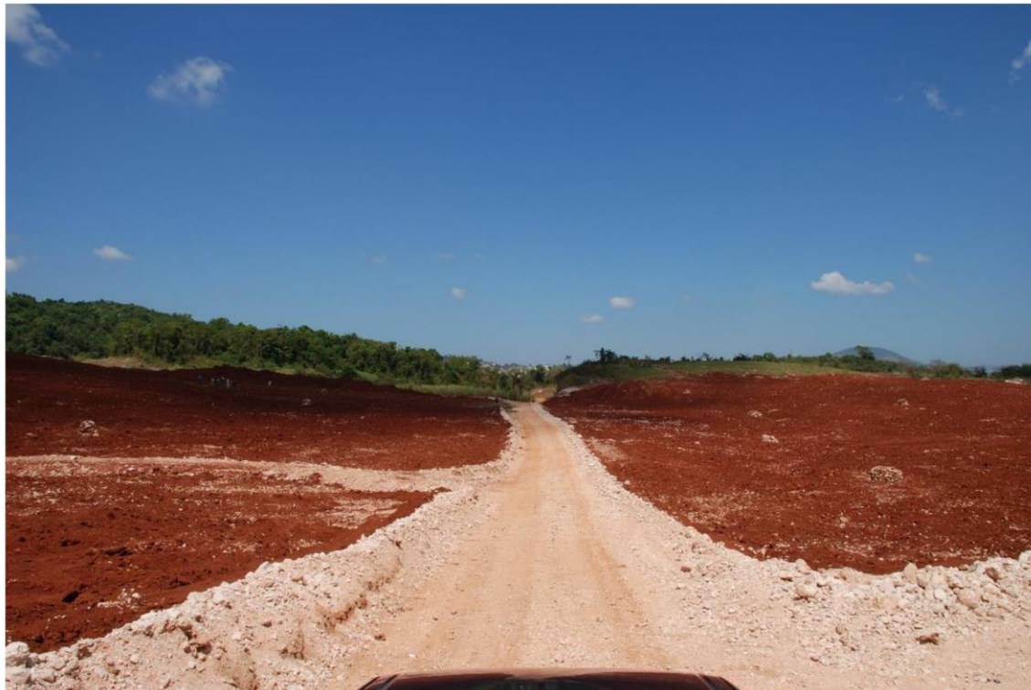
Figure 8-4: Restoration process – top soil placed (Manchester)
