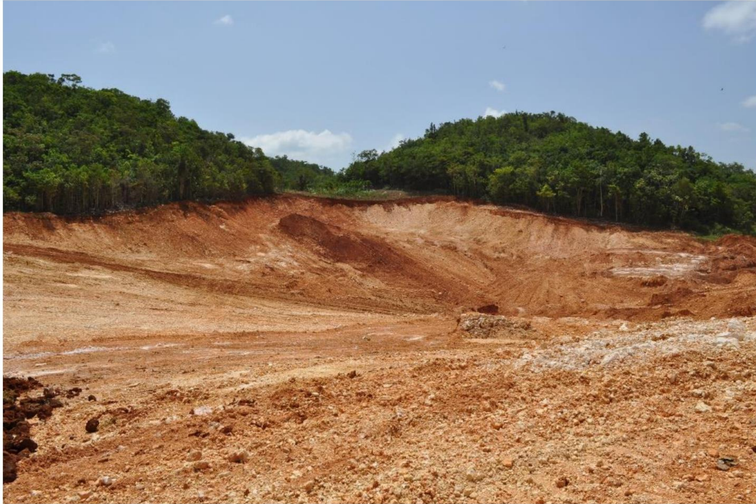
Figure 8-1: Mined out pit being leveled for reclamation and restoration
