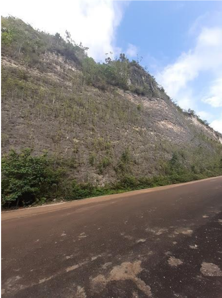
Figure 5-90: Section view of roadway cut through a hillock
