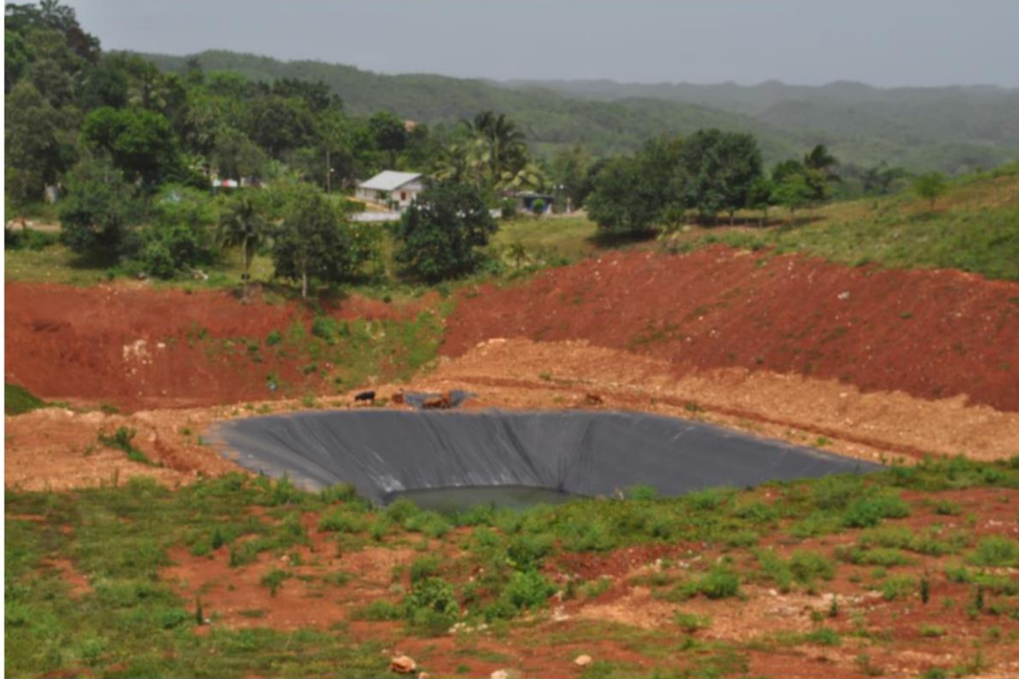
Figure 8-15: Water catchment at greenhouse project site – Clapham, St. Ann
