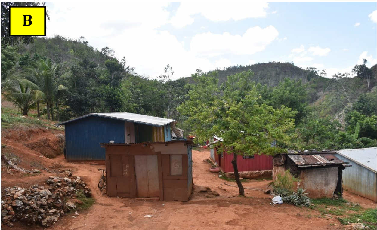
Figure 5-57: A - Derelict occupied house in the south of the SEPL 524 | B - Unplanned development in close proximity
