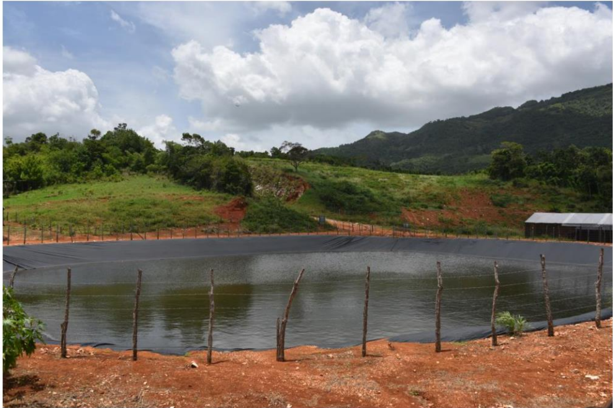
Figure 8-18: Water catchment at greenhouse site – Blue Mountain, Manchester
