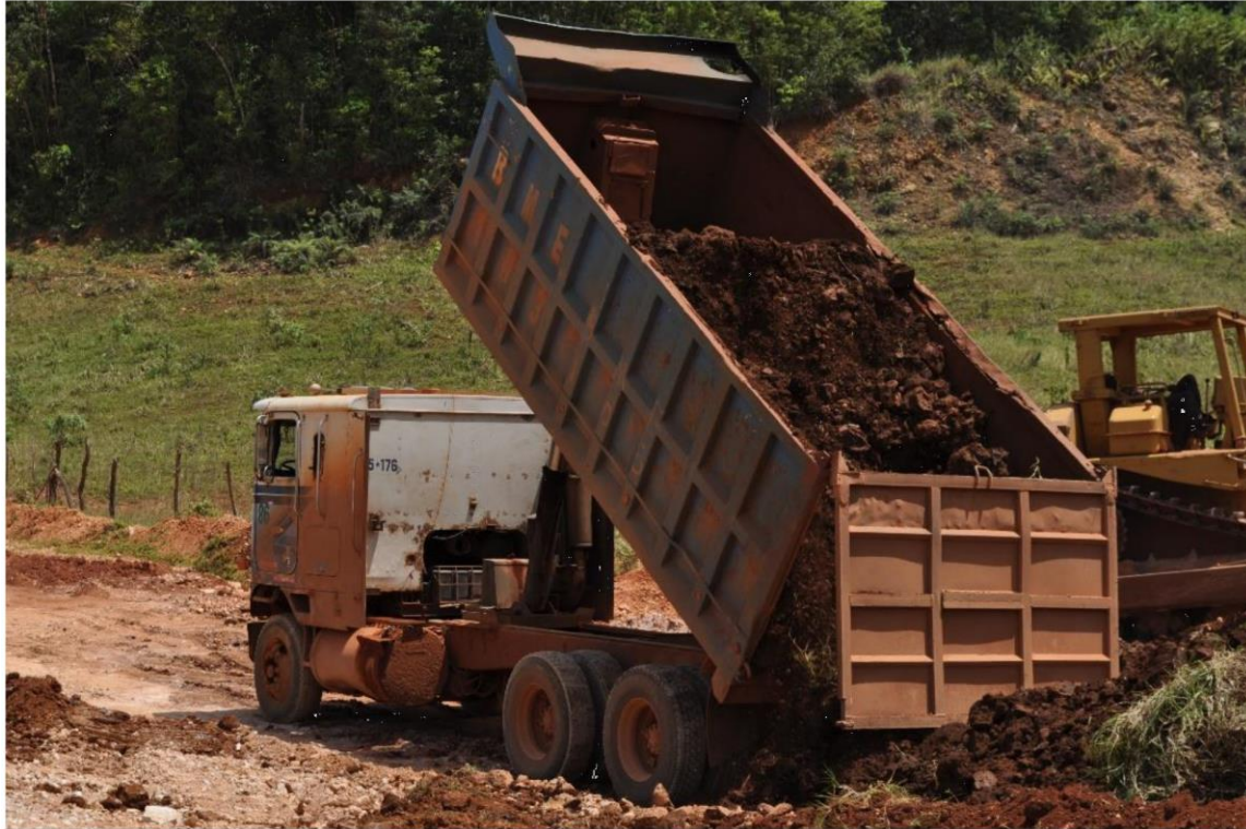
Figure 8-3: Top soil hauled for use in the reclamation process
