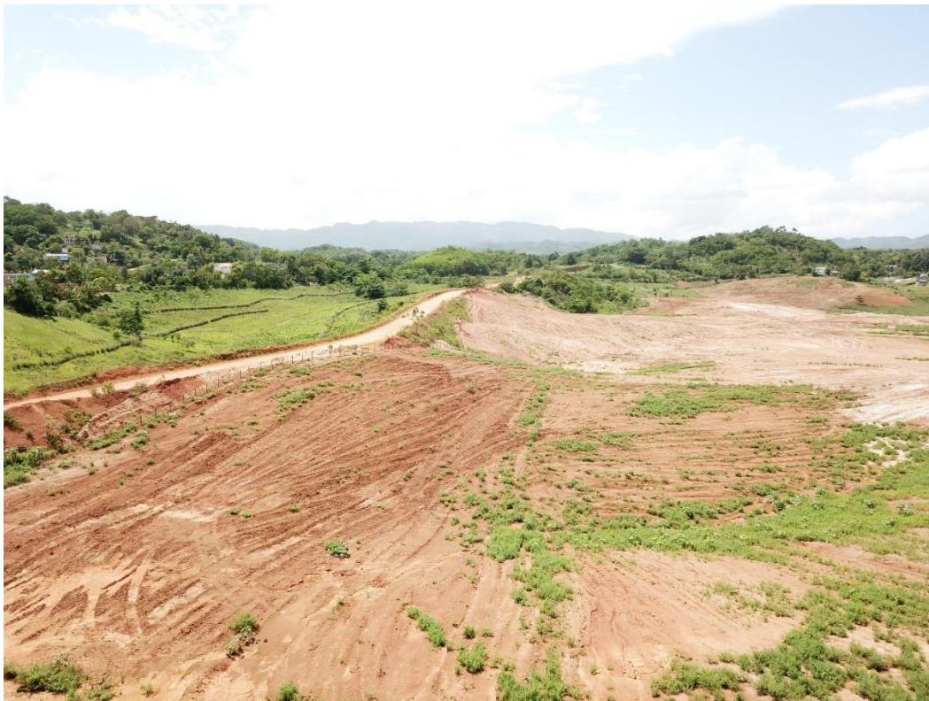
Figure 5-191: Rehabilitated mine at T24
