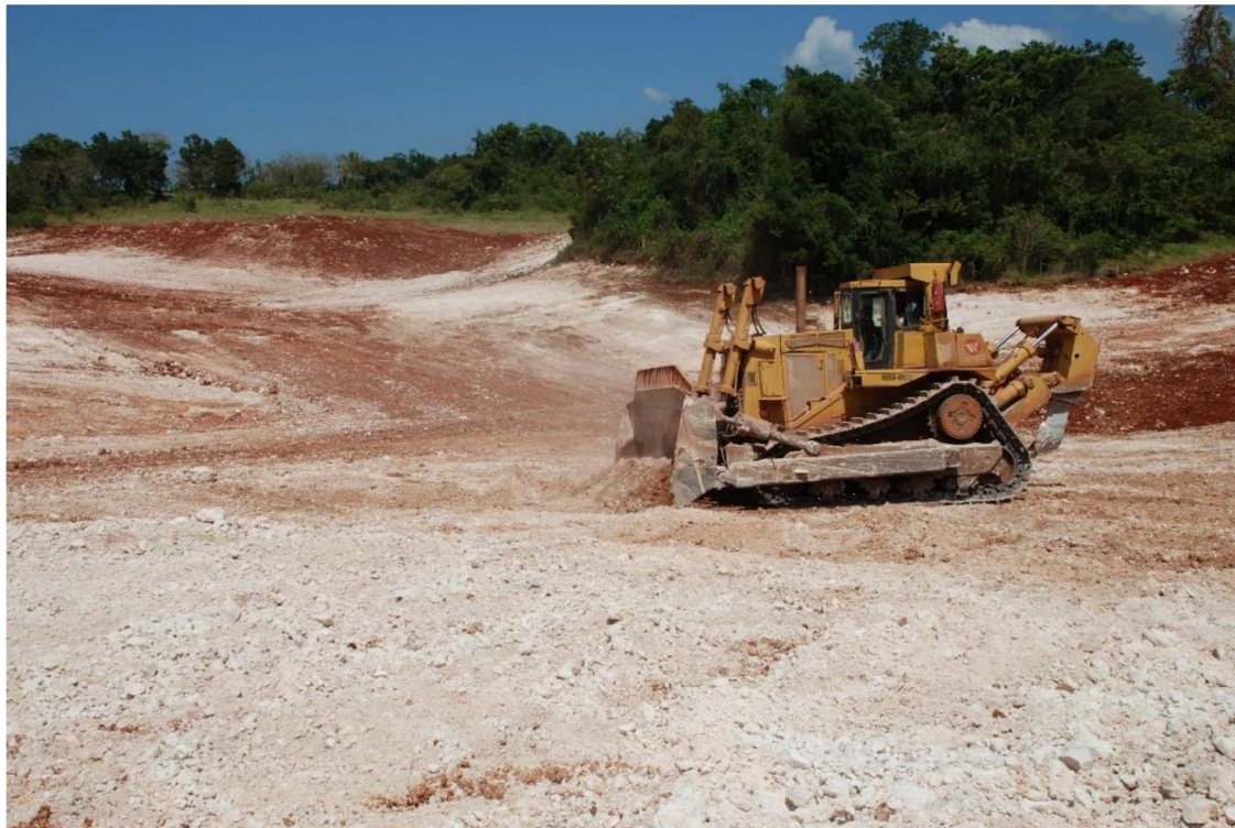
Figure 8-2: Reclamation Process – Contouring and Landscaping (Manchester)
